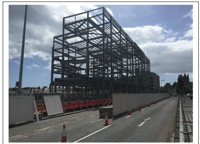
Exeter street lane closure commenced.
