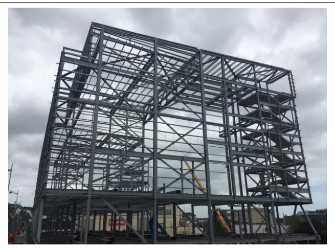
Steelwork installation ongoing to Zone 5.
