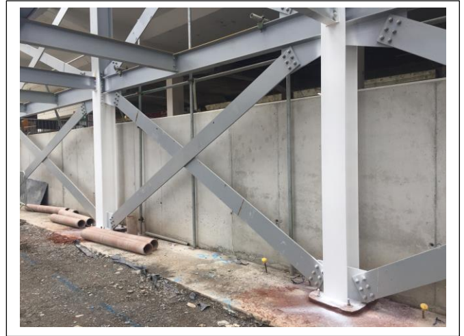
Intumescent painting commenced to structural steelwork
